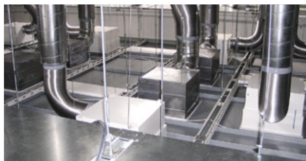
clean-tek system with split-level ceiling
