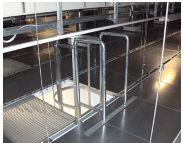
ceil-tek ceiling systems can be walked-on
