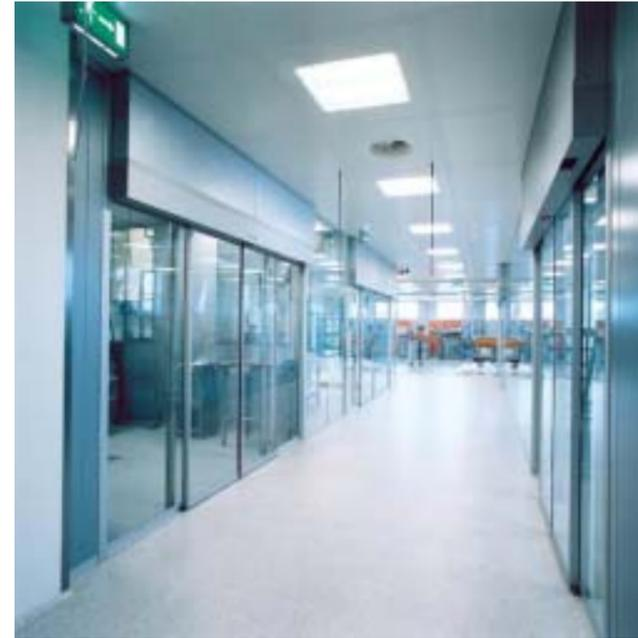
In narrow production aisles, automatic sliding doors are the ideal alternative to revolving doors. The leaves automatically open to their full width and materials can be transported without the leaves getting in the way. The leaves are electronically monitored to prevent unwanted closure.
