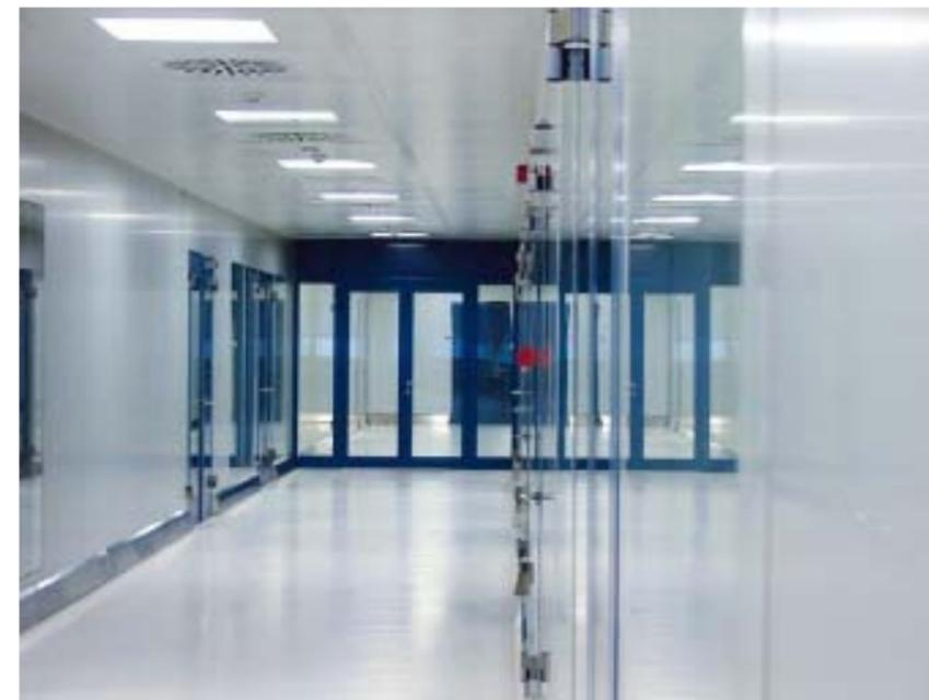
The modular design enables quick and easy replacement of the modules, e.g. in the event of severe damage or also during alterations.
