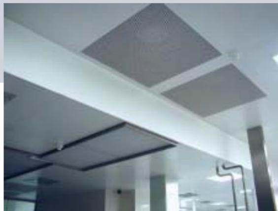
For every ceiling system **clean-tek** offers appropriate lights with different configurations. All lights have a glass cover with a translucent sanded surface as standard. With walk-on ceilings, the lights are also walk-on.
