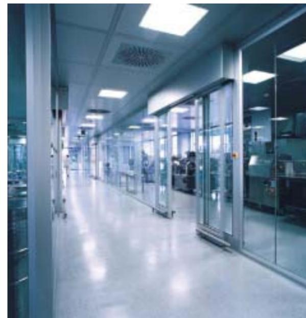
**clean-tek** builds F90 fire walls for room heights of up to 5,500 mm with one or two-sided GMP cladding. F30 glazing can also be fitted into these walls flush on both sides. There are likewise F30 door units that are tailored to the system with glazing that is flush on both sides.
