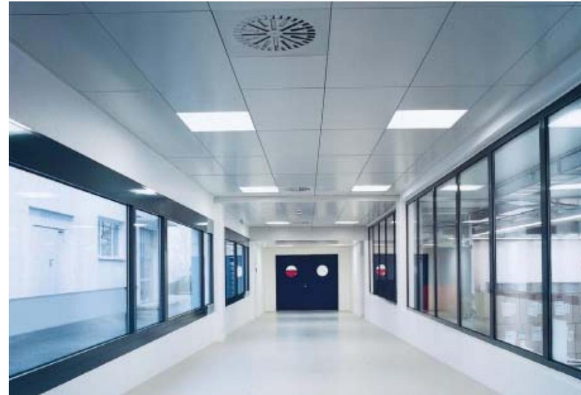
**clean-ceil** is the perfect rational solution for single-skin, non walk-on grid ceilings. Particularly flexible, particularly easy to assemble, particularly economical. This recently developed ceiling system is based on the experience acquired through developmental refinements made over many years and meets all the requirements for clean rooms of the widest range. The standardised grid size means that all the ceiling modules can be delivered from stock with the shortest possible leadtimes.
