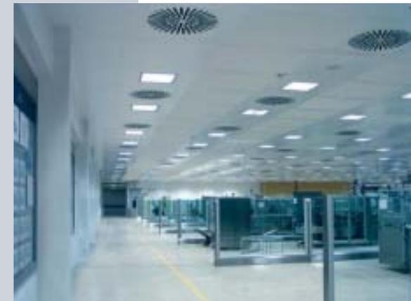
All the function elements are fitted from the clean room side and are easily accessible from below. Therefore very restricted ceiling cavity heights are not a problem either.
