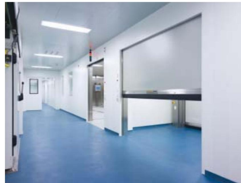
Cutouts can be made at any place in the wall you require, even if they involve several modules due to the size. All **clean-tek** wall modules can be altered or removed at any time, without any special tools, and they can also be replaced if needs be. As is appropriate for a flexible walling system. In addition, the construction system also enables compensation of dimensional tolerances. Joints with walls and ceilings are made with vibration isolation.
