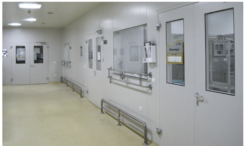
Combination of ramming protection at floor and wall levels as a custom-built installation
